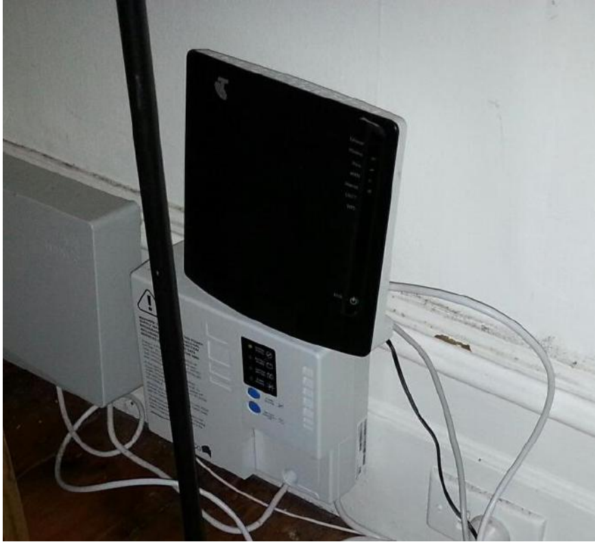
Figure 3 – Photo of internal equipment
