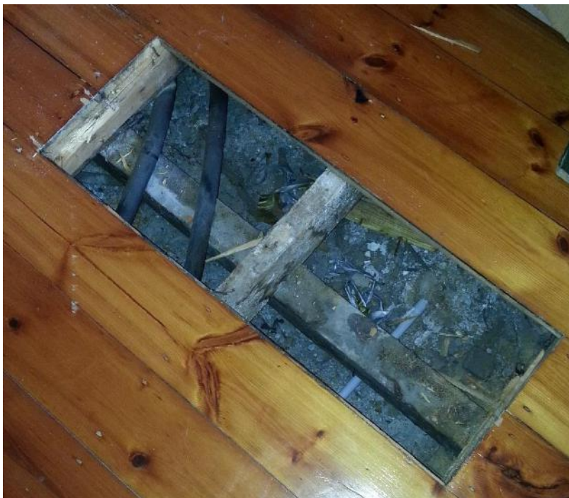
Figure 7 – Hole in lounge room floor boards.
