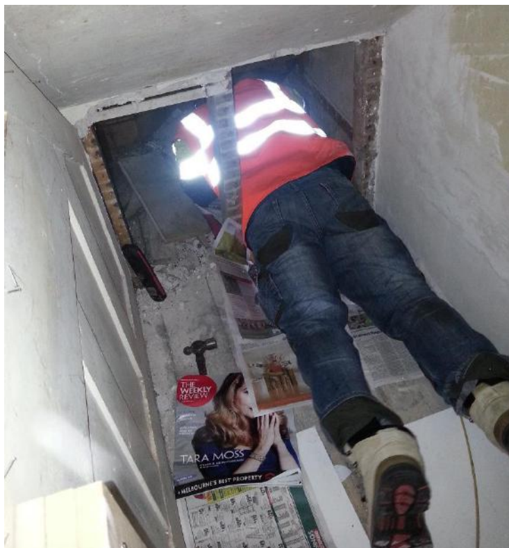
Figure 9 – Cramped access to the hole in floor boards beneath stairs.
