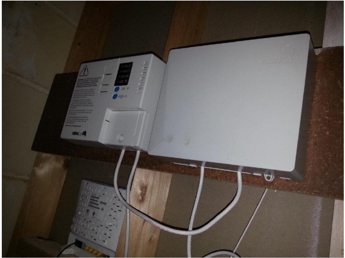
Figure 10 – NBN equipment beneath the stairs.
