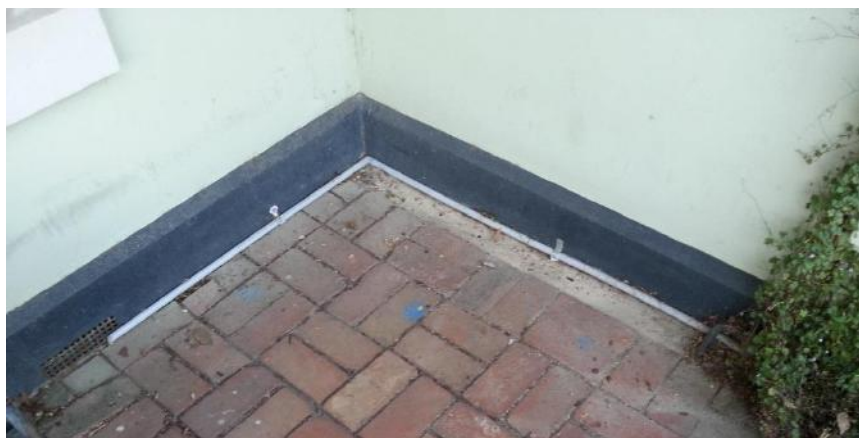
Figure 2 – Photo of conduit on front veranda. A corner of the white NBN Utility box can be seen on RHS behind the fairy fern that we planted in an attempt to reduce the visibility.
