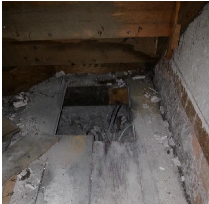
Figure 8 – Hole in floor boards beneath stairs.
