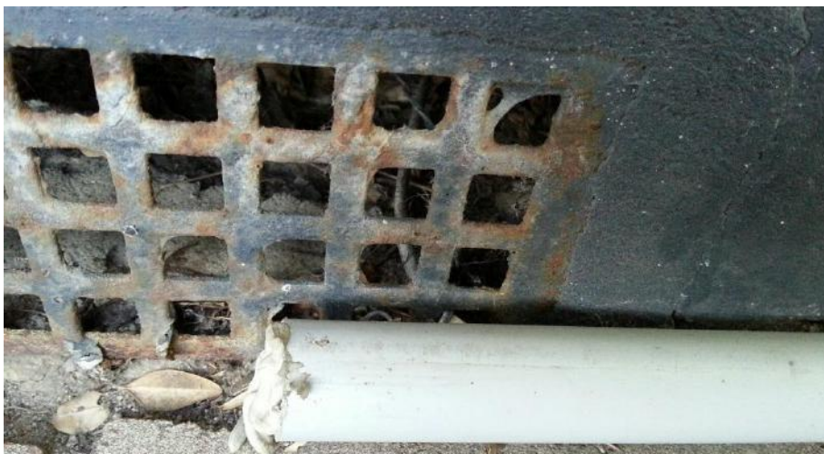
Figure 4 – Close-up photo of exposed conduit and unprotected optical fibre passing through sub-floor vent
